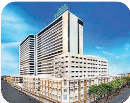
SIR HN RELIANCE FOUNDATION HOSPITAL, MUMBAI
